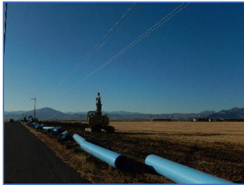
Pipeline installation near Arco
