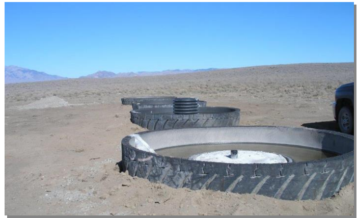
Each trough holds 1,500 gallons
